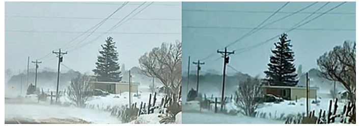
These are photos from video clips of lines galloping in EEA service territory. The photos are less than half a second apart. You can see the conductors near the top of the photo have moved from overlapping to being several feet apart. Photos courtesy of Matt Larsen.
