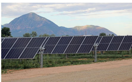
▲ The Montezuma solar generator delivers 5 megawatts of capacity and utilizes single-axis tracking to follow the arc of the sun to maximize energy production. It produces enough energy to supply over 1,600 homes for an entire year. Photo by Denise Moore, EEA
