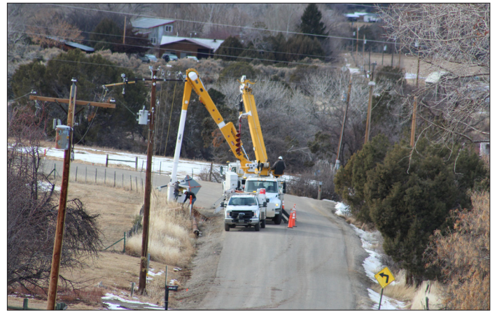
▲ An EEA linecrew upgrades a distribution line on Road T.5 earlier this year.
